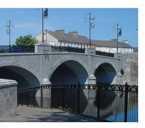
The resulting brand new bridge retains both the character and beauty of the old bridge. The remodelled structure carries in the region of 21,000 vehicles on a daily basis. This landmark bridge has been widened from 16.1m to 22.2m, which has led to the creation of two lanes of traffic and a cycle track in both directions.
